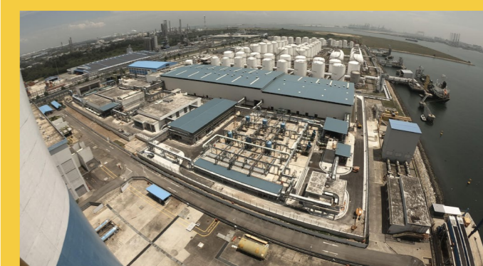
Jurong Island Desalination Plant (JIDP) (credit to Tuas Power)
