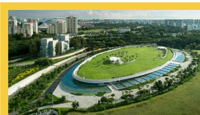
Keppel Marina East Desalination Plant (KMEDP) KMEDP is Singapore's first large-scale dual-mode desalination plant capable of treating both seawater and freshwater. It features an innovative design to incorporate underground treatment facilities and has an open green rooftop space for recreational activities.
