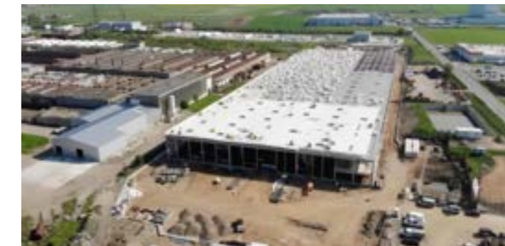
Câmpia Turzii Industrial Park, Cluj county Source: https://turdanews.net/
