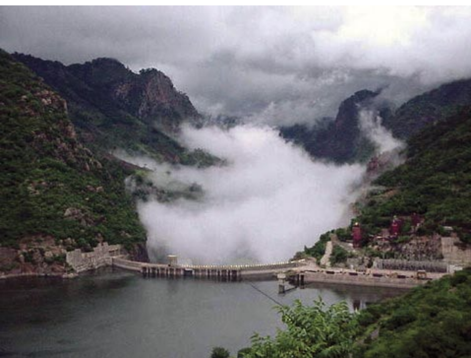
Cahora Bassa Hydroelectric Dam, Tete Province
