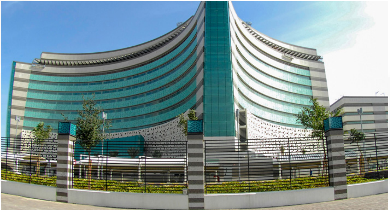
Jaber Al-Ahmad Hospital is the largest hospital in the Middle-East region 2018
