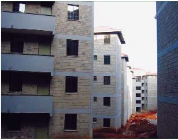
Construction at Kibera decanting site
