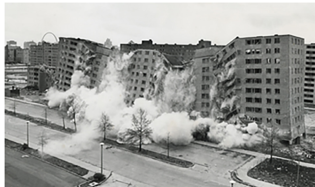
Figure 17: Pruitt-Igoe: failure of the modern, direct supply approach
