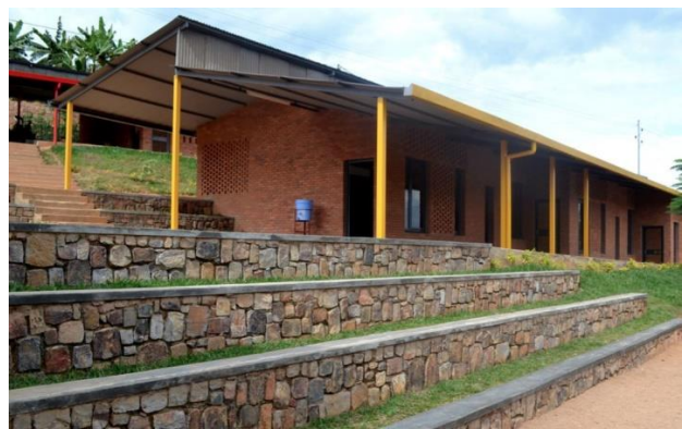
Ecole primaire d'Umubano au Rwanda, Arch. MASS Design Group. Source photo: Google
