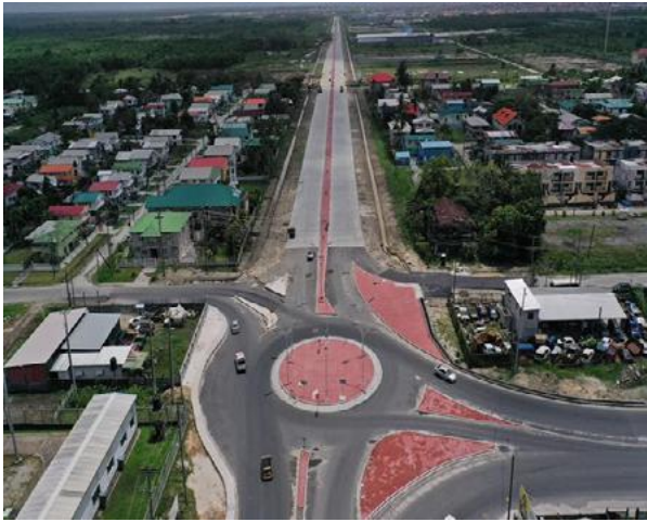
Figure 40: Overview of the Mandela to Eccles Highway and roundabout
