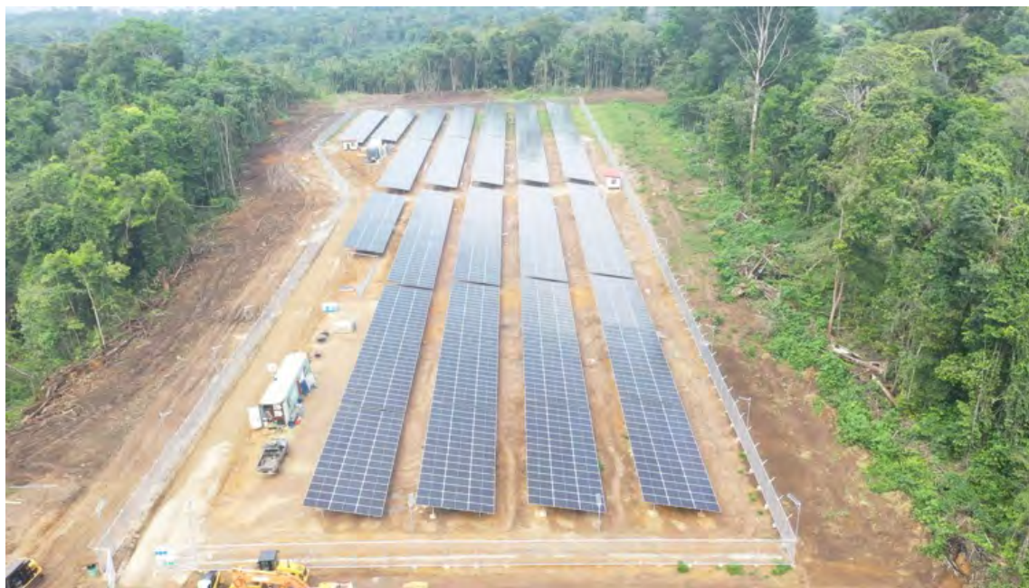
Figure 17: 1.5MW Solar Farm at Bartica, Region 7
