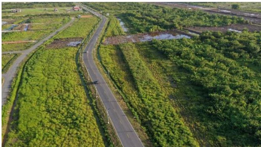
Figure 42: Overview of Eccles to Great Diamond, East Bank Demerara Interlink Road
