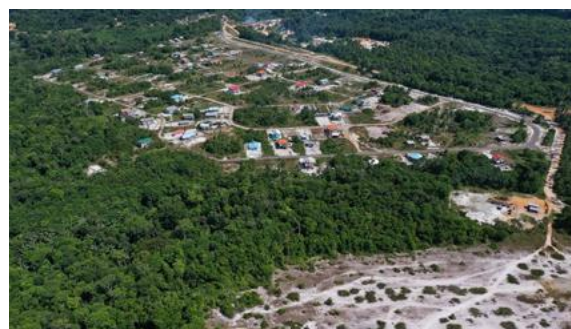
Figure 37: Clearing of 120 acres of land for Bartica Housing Project
