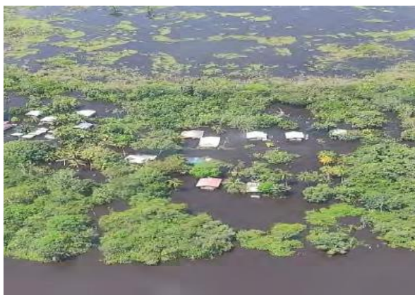
Figure 51: Aerial View of 2021 Flooding in Kwakwani, Region 10
