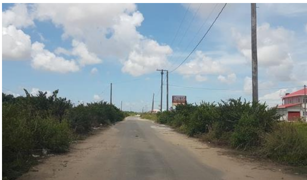
Figure 12: Access Road from Herstelling to Prospect constructed of Asphalt
