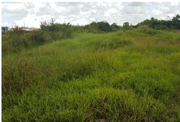
Figure 4: Silted Up Main Drainage Channel Adjacent to Project Site (2020)
