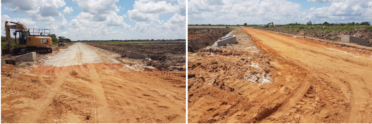
Figure 14: Construction of Access Roads Adjacent to the Site
