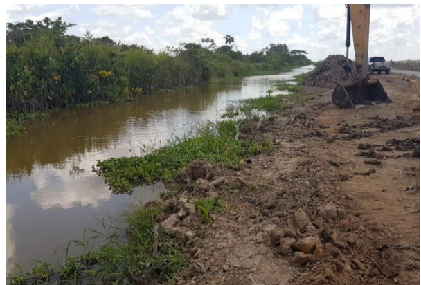
Figure 5: Cleared Main Drainage Channel Adjacent to the Project Site (October 2021)
