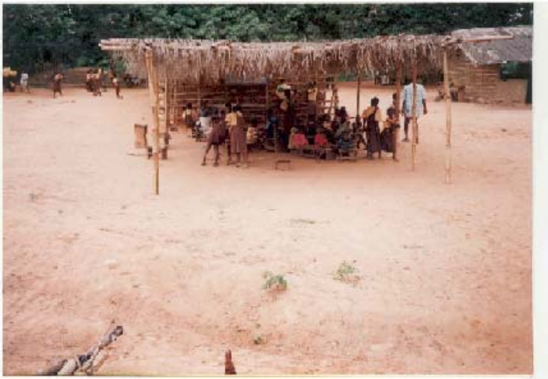
A Primary School structure
