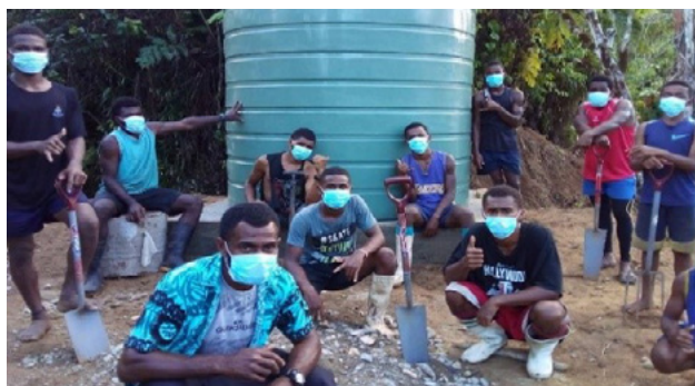
Water system successfully installed by the villagers of Naqarawai, Namosi. This was done during the COVID-19 lockdown. PC – Laisenia Tui. (Source: WISH Fiji, Fiji National University)
