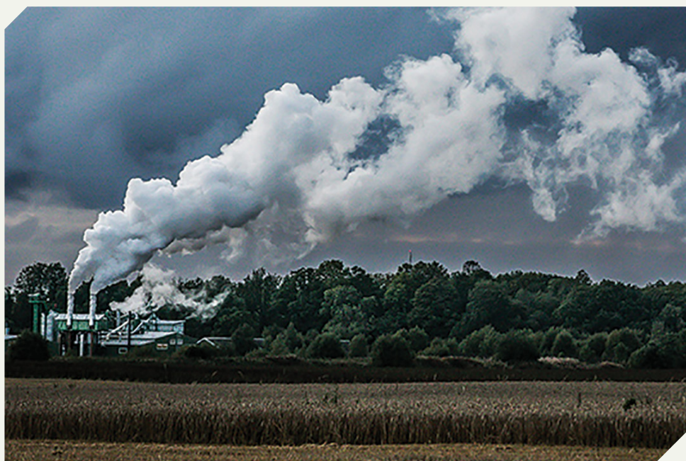
WARMESTON PELLET PLANT IN PURILA
