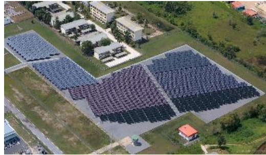
Aerial view of the TSB plant
