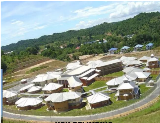
Welfare Home Complex in Belimbing
